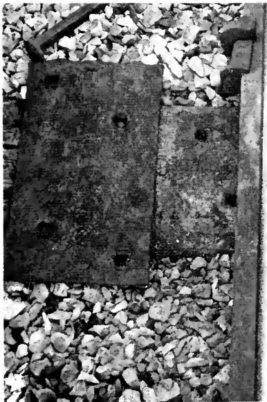
Fig. 11. South Portion Section 46, 14-in Racor Tie Pad, Coated, After 32-months' Service in the Inner Rail of the 5° Curve Little sand, fair seal, 80 percent coating left on tie, pad in good condition.
